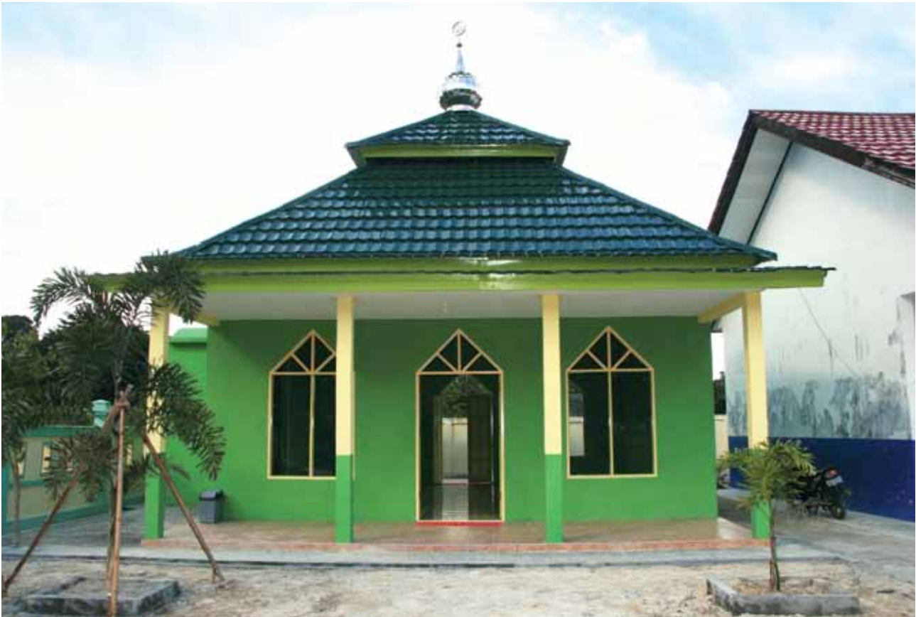
Musholla construction at SDN 001 Saliki, East Kalimantan.
