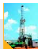
Rig 14 Ogan Ilir, South Sumatera
